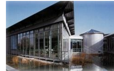
Zuken GmbH European Headquarters Munich, Germany
